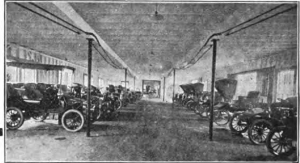
Interior view of Auto Garage.
